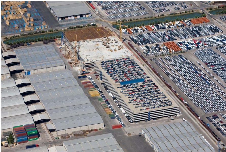
Photo 1: Construction of the new vehicle warehouse
