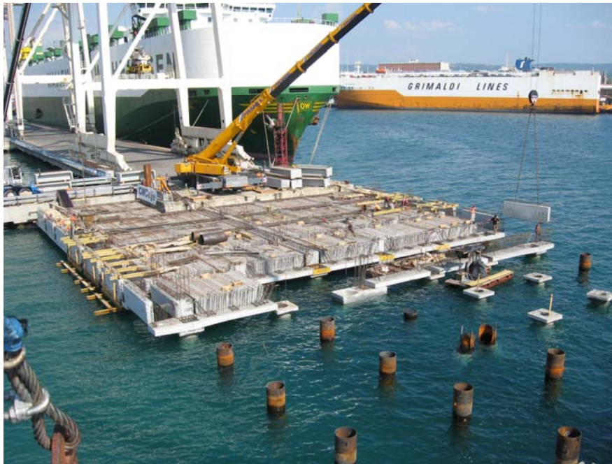
Photo 2: Construction of the extension to Pier No. I
