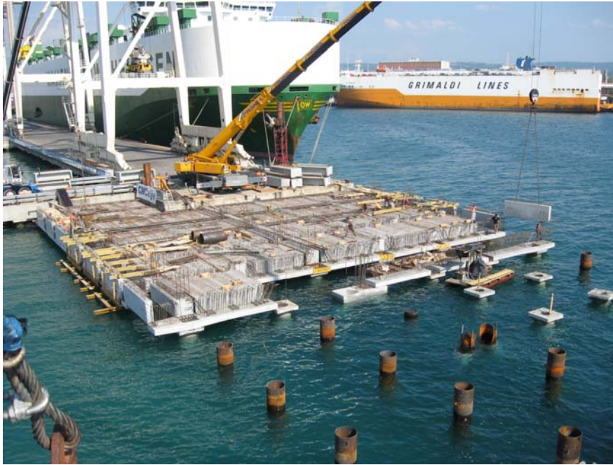
Photo 2: Construction of the extension to Pier No. I
