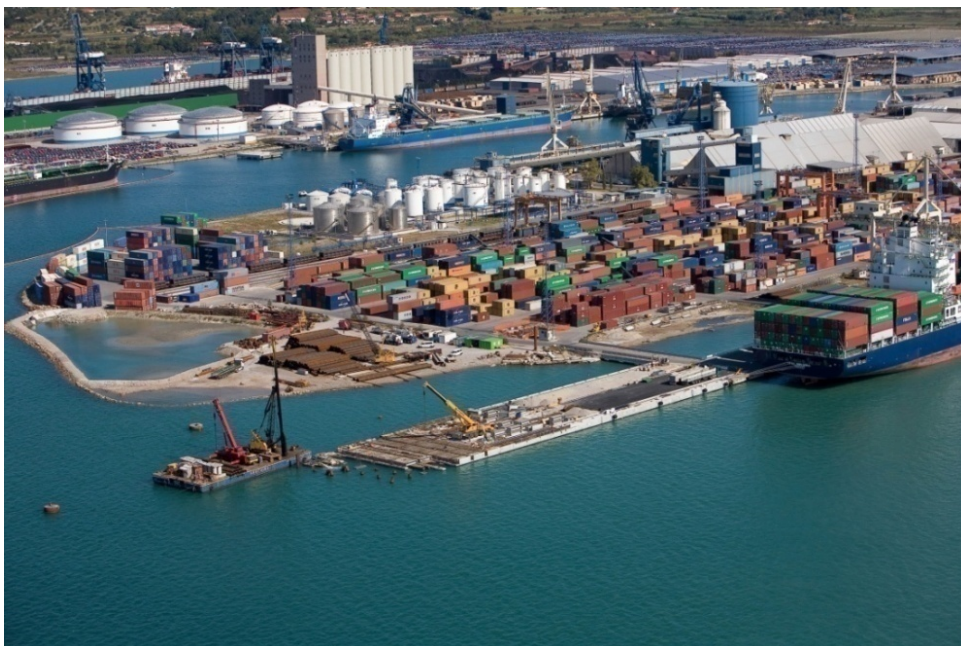
Photo 2: Construction site for the extension of Pier No. 1
