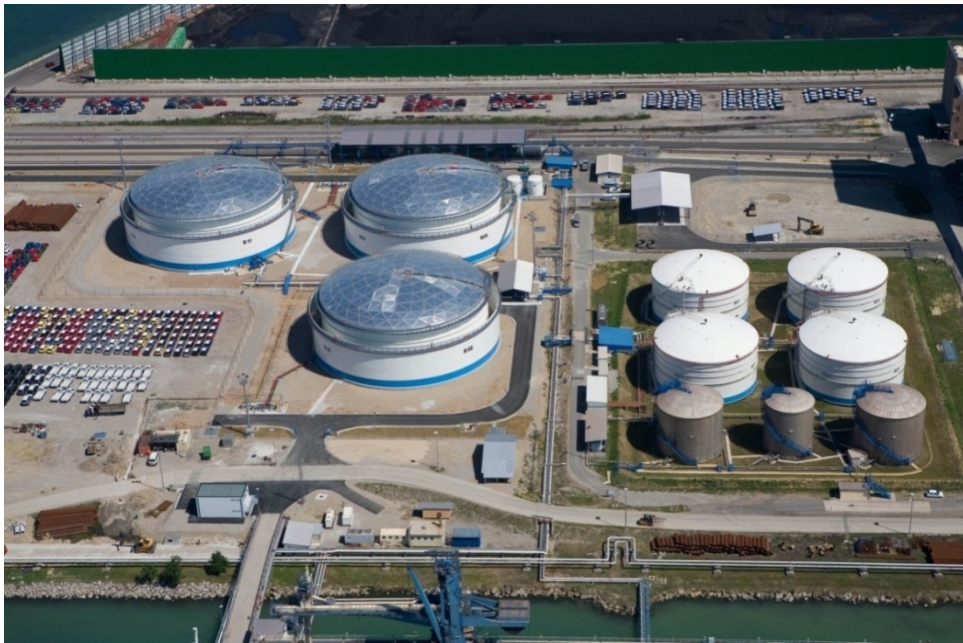
Photo 1: New oil derivatives storage at the Liquid Cargo Terminal
