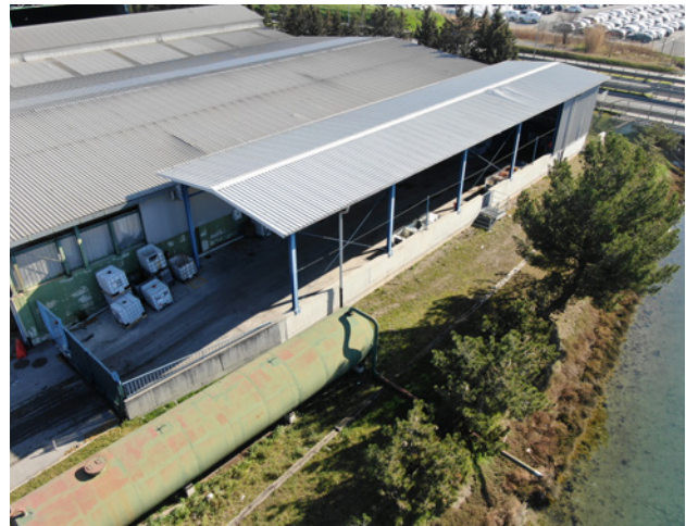
Waste Management Centre – hazardous waste storage facility, Photo: Matevž Bregar
