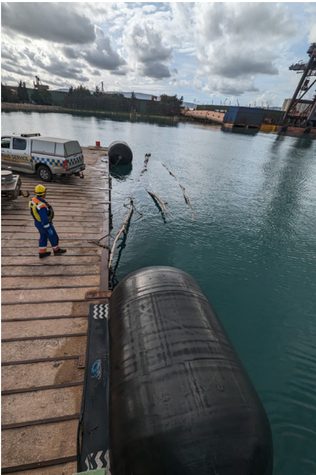
Figure: A view of the cleaning of debris throughout the Luka Koper, d. d., port water area and the installation of spill socks in the Basin II.
