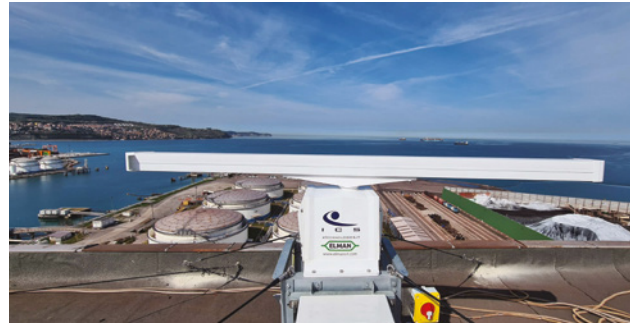
Figure: A radar for detecting pollution at sea, installed on the roof of a silo of Luka Koper, d. d. Photo: Jure Barovič
